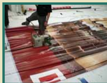
Track Welding on Floor
